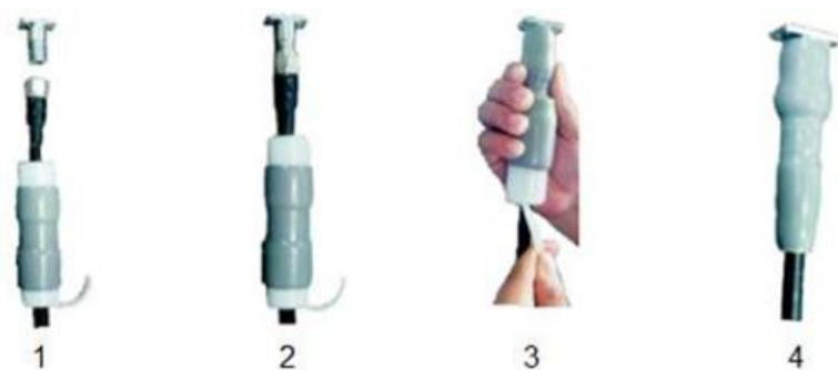
Figure 2-2: Weatherproofing
